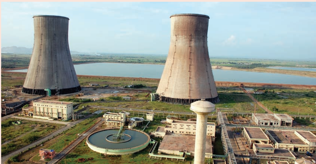
Ballari Thermal Power Station
