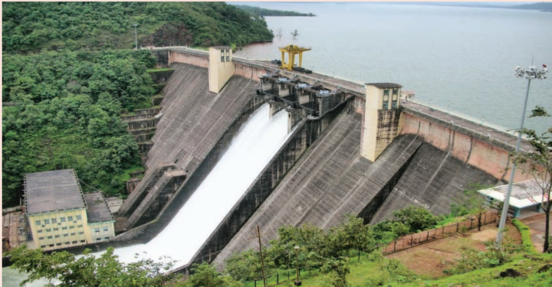
Supa Dam, Kali Project
