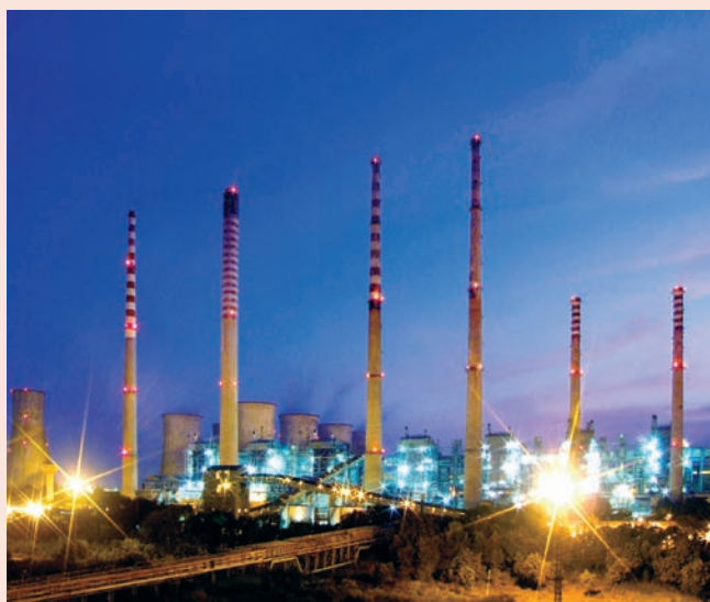
Raichur Thermal Power Station
